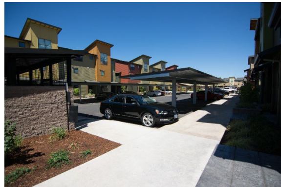
Off-street parking typically includes driveways, surface parking lots, and parking garages.
