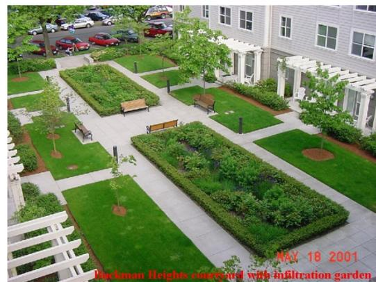
The Presumptive Approach shall be used for all other water quality, flow control and flood control designs in conjunction with a measured infiltration rate. Rain gardens shall be designed to pond water for less than 30 hours after each storm event.
