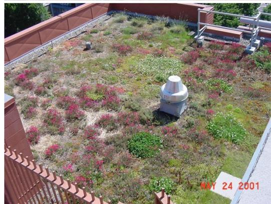
different strengths and functional characteristics. Some of these products require root inhibitors and other materials to protect the membrane. Numerous companies manufacture waterproofing materials appropriate for Eco-Roofs.
