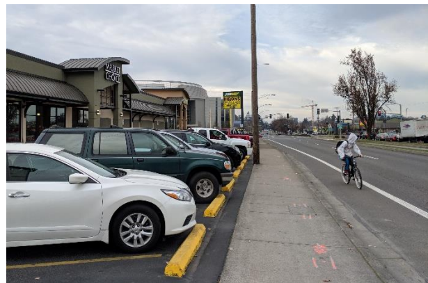
Sidewalks without a buffer and standard bike lanes are not comfortable places for people to walk and bike on Franklin.
