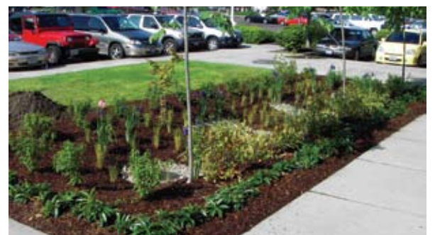
This landscaped area at Oakway Center is actually a stormwater treatment system that functions much like a wetland, filtering stormwater that flows into it from sidewalks and parking lots.
