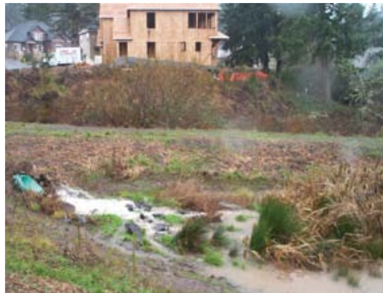
Rain carries loose soil from a construction project into the stormwater system. This muddy mess will make life difficult for salmon eggs (left) and other creatures downstream.
