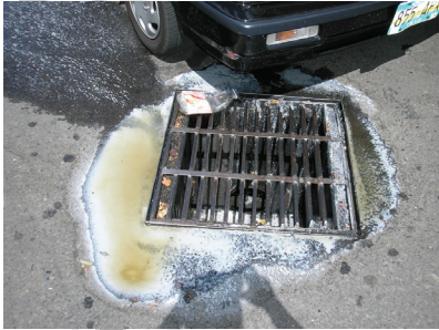
Pollutants entering an unprotected storm drain are carried directly to local waterways.
