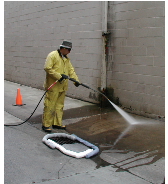
Following best management practices (BMPs) and protecting storm drains will help keep pollutants out of local waterways. See the back of this sheet for more details.
