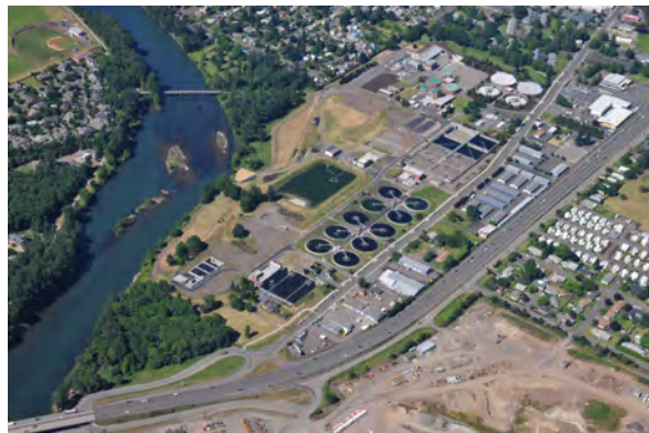
Regional wastewater treatment facility on River Avenue in Eugene
