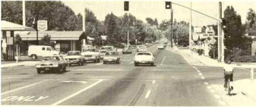
Busy arterial intersection (ADT 34,000) was recently widened to 66 feet to provide needed center-turn lane plus bike lanes on 4½-foot-wide concrete gutters.**
