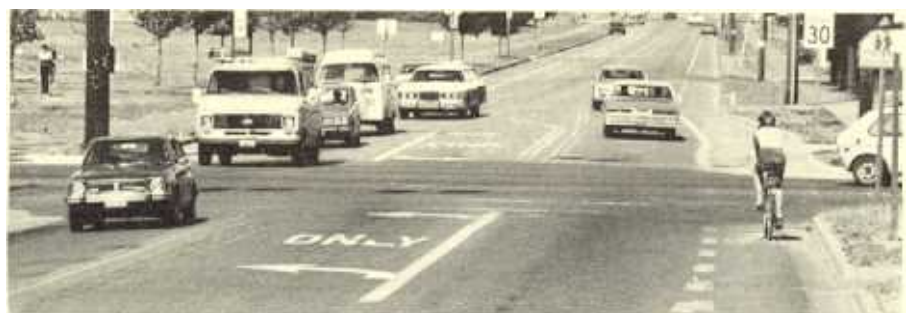
At intersection of a collector and an arterial street (average daily traffic, 21,000), a Junior High School and retail shops attract bicyclists. Special widening and parking removal on the collector street made space for curb-side bike lanes.* *
