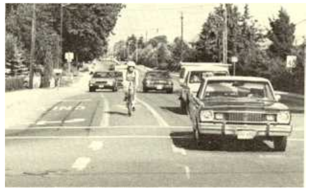
Right-turn bay at widened intersection. Motorist and bicyclist cross paths in advance of intersection.
