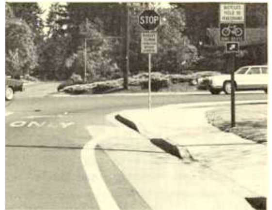
Sidewalk ramps may help cyclists "cut the corner" when turning traffic is heavy.
