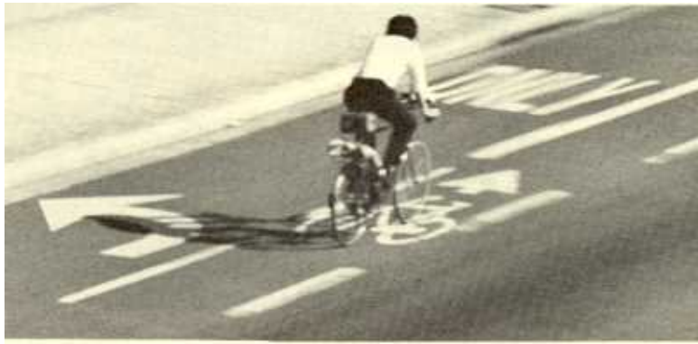
Bike lane continues straight on one-way street when parking lane becomes left-turn only lane.
