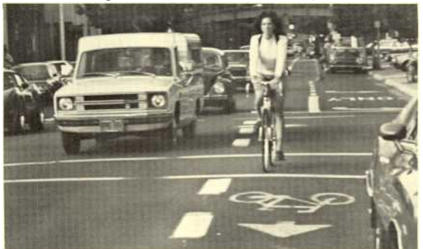
Bicycle symbols, directional arrows, and wide stripes claim the space. The stripe is dashed through the intersection.
