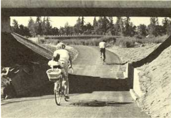
Railroad underpass , completed just in time for Olympic Trial Marathon in 1972, provided access to river bank trails.
