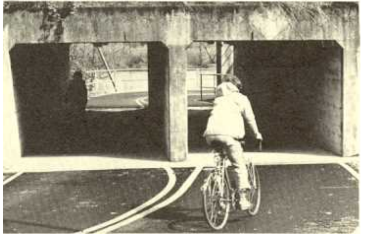
Innovative design turns abandoned culverts into efficient bike tunnels beneath the railroad.
