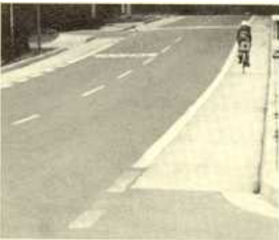
Wide, concrete gutters make a smooth, unbroken riding surface (above and center).
