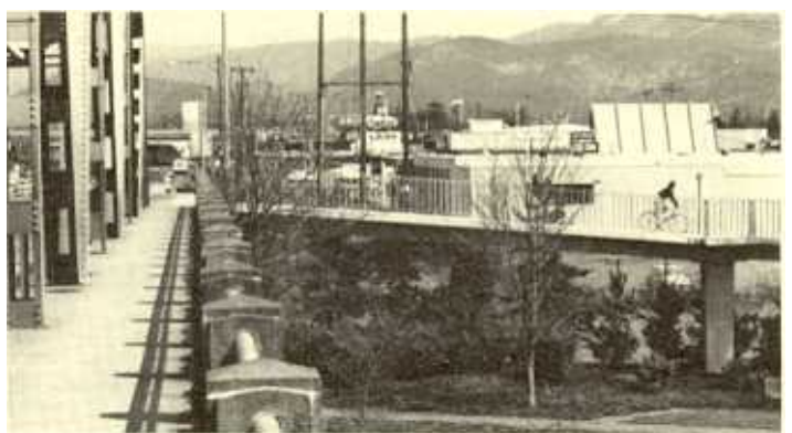
Ramp carries cyclist from bridge to riverbank trail.
