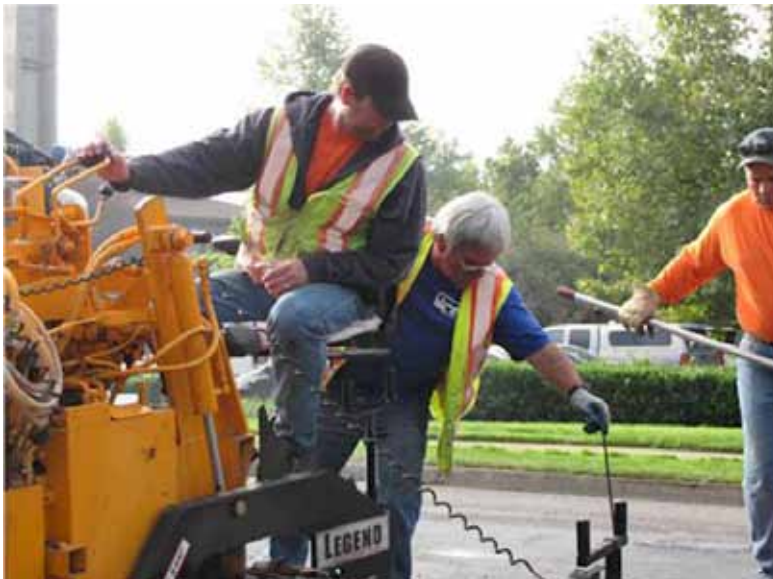
Paving crew constructs maintenance overlay
