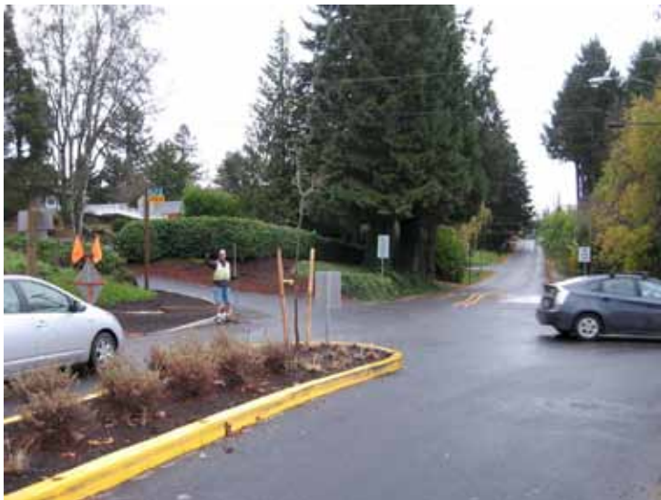
Crest Drive improvement project
