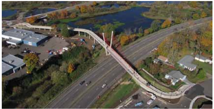
New Delta Ponds multi-use bridge
