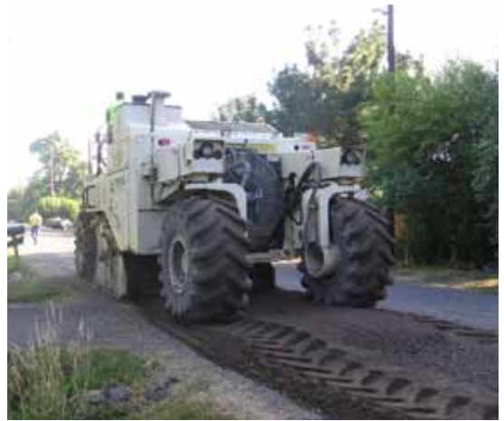
In-place street recycling on Riverview Street
