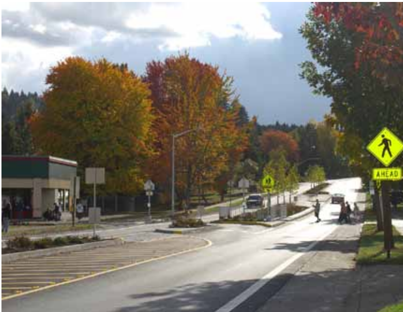
Bailey Hill Road project won a state safety award
